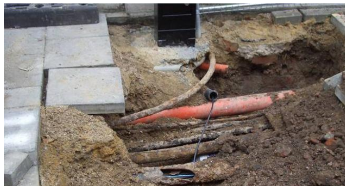
Figure 2 – The Challenge Below the Surface (courtesy of TfL)
